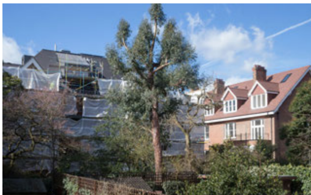
▲ 14 Netherhall (left) as seen from Maresfield: the roof of the additional storey dominates Otto Schiff House
