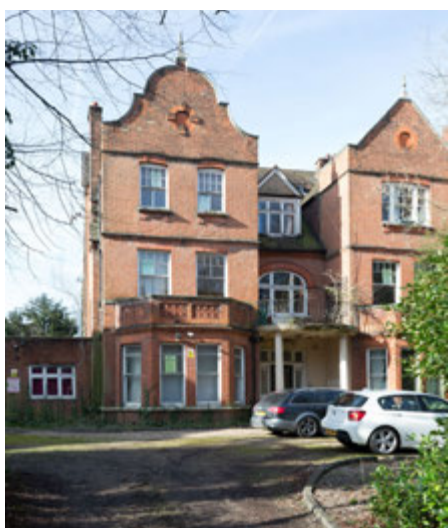
▲ 13 Netherhall Gardens, one of the few original large houses in our area, now for sale and redevelopment.
